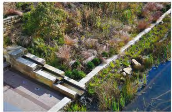
ABOVE A trough that descends the hillside doubles as a design feature and an oxygenation device that cleans and aerates water pumped up from the tropical lagoon.
