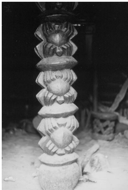
Fig. 4. Carved trunk of Prunus africana used as a center pole to support a roof.
